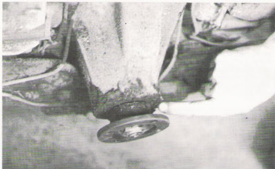
With the axle on the floor, a look around the propshaft flange shows that the oil seal has been leaking for some time. The drive shaft output flanges are also moist so oil will have been issuing forth from here as well. The obvious danger is oil spraying on the inboard disc brakes.
